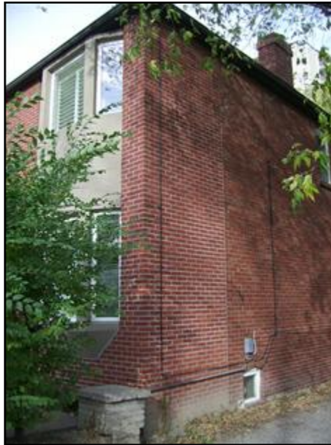
9. West addition - Southwest corner
