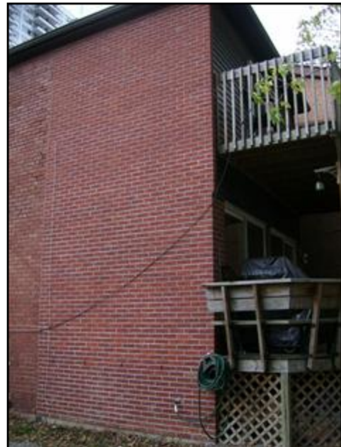
8. East Addition - Southeast corner
