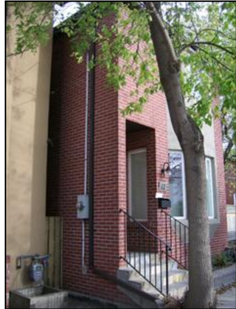
6. West Addition - Northwest corner
