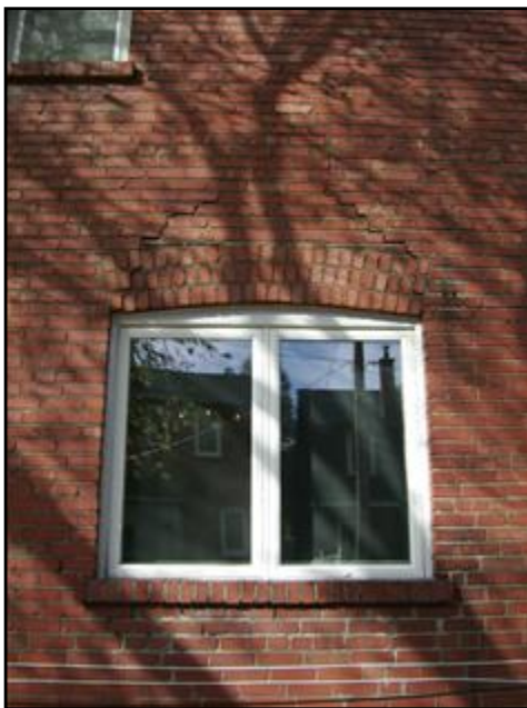
15. South wall - First floor arch
