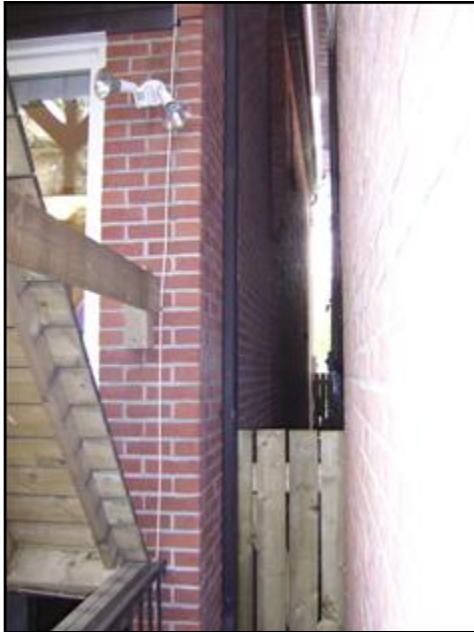
5. East Addition - Northeast corner
