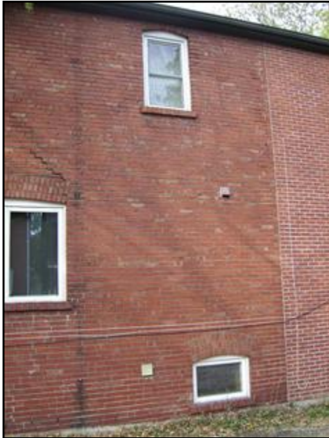
10. South wall - East end
