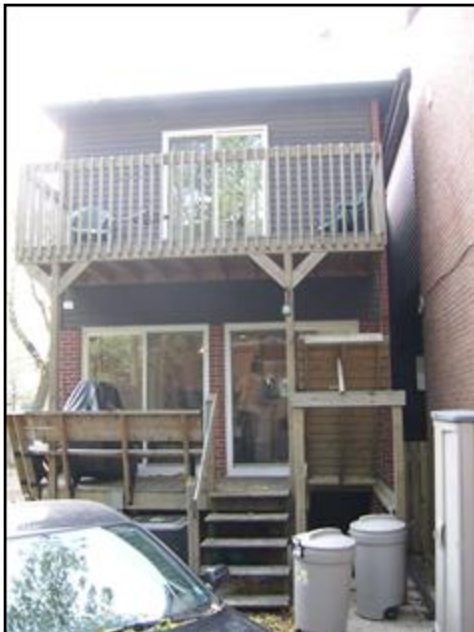
7. East Addition - East wall
